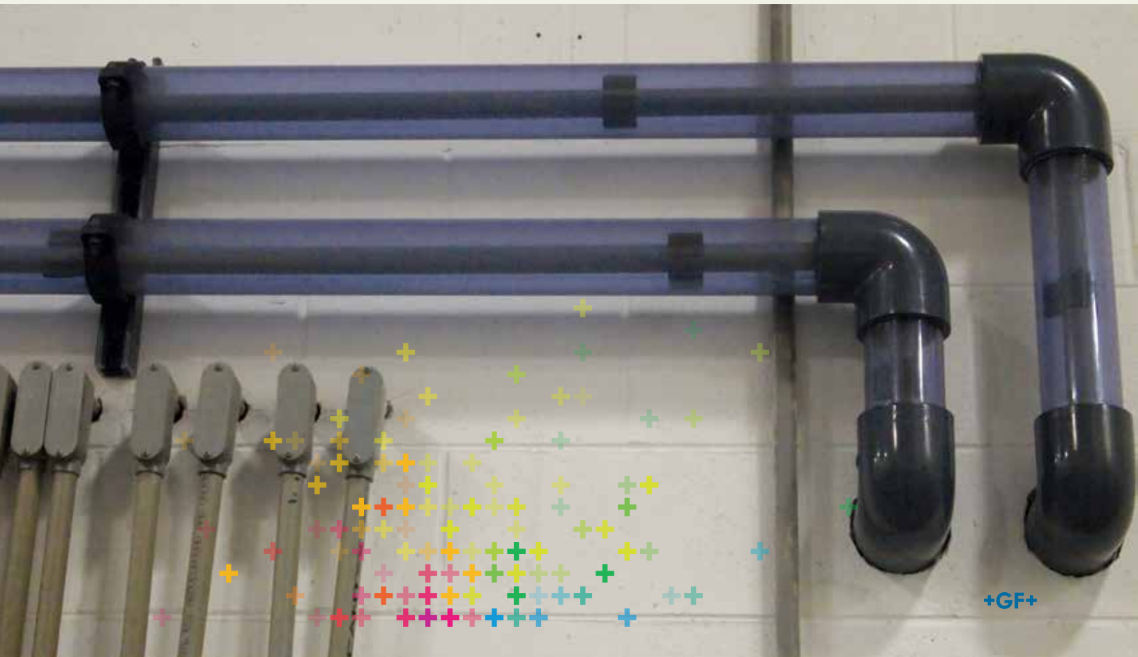
Closure coupling installation
